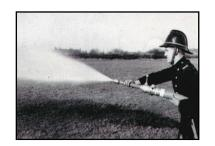
**2.** Branchpipe control adjusted to water spray position
